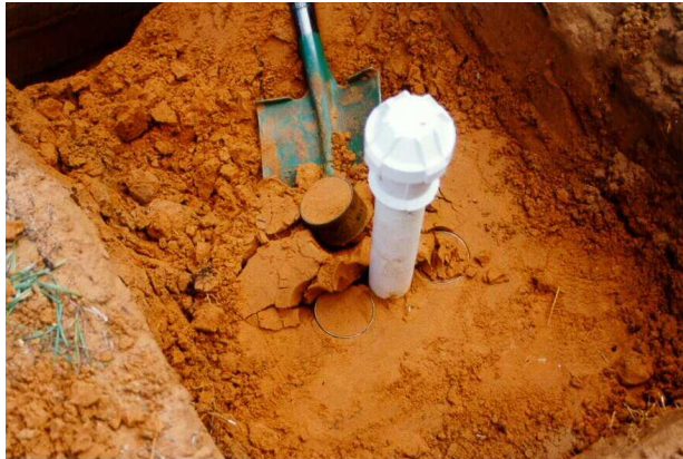
Photo 8. Removing sampling rings
