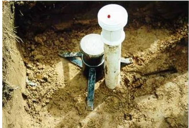
Photo 6. Placing ring extension on top of ring
