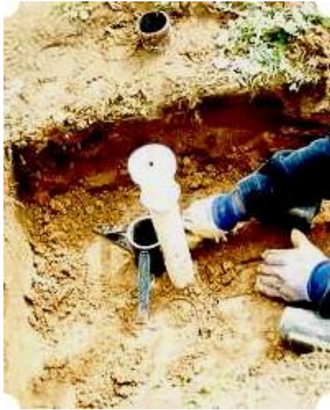
Photo 5. Placing top on ring extension ready to hit with mallett
