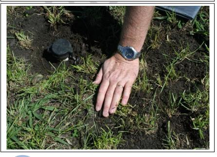
Fill the cable trench with soil and compact down.
