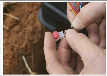
Squeeze Scotch-Loks<sup>®</sup> firmly to ensure good connection.
