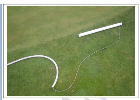
To pull probe cable through conduit simply attach probe cable to "Pull-Wire" of the conduit.
