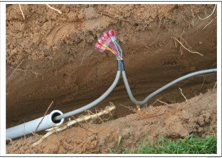
The completed cable join between DTU cable and Probe cable.
