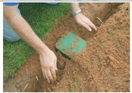
Continue burying cable in conduit and connect cable terminal to DTU.
