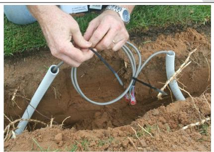
Ensure excess cable for servicing is left in a loop at the joining point of DTU cable and probe cable.
