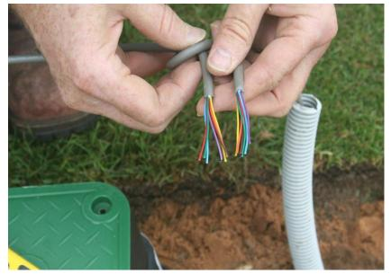
Position the cable leading to the probe and cable leading to the data transmission unit next to each other. Ensure that the cable leading to the DTU is also protected by conduit.
