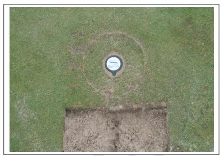
Refill the trench and smooth the surface with shovel. Connect the probe cable to the DTU.
