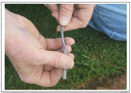
Remove 50 mm of cable sheath.
