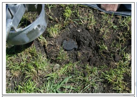
Centralize the grass sod around the Flat Cap.
