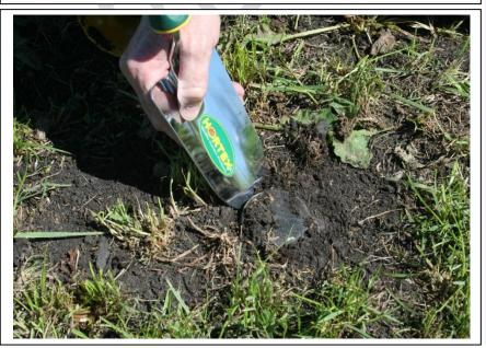
Use small hand trowel to remove loosened soil around the Flat Cap.
