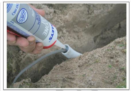
Allow enough cable to make a loop so that maintenance of the probe can be done at a later date.
