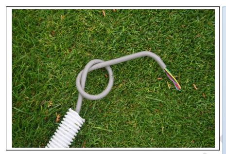
Secure the end of the probe cable with a knot. Before laying the conduit and the cable into the trench, proceed with the installation of the probe access tube.
