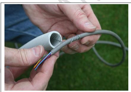
Pull the probe cable through using the "Pull-Wire" at the other end of the conduit.
