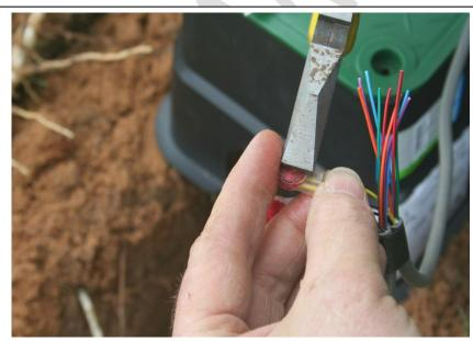
Inspect each Scotch-Lok® to ensure wires are connected and have not slipped.
