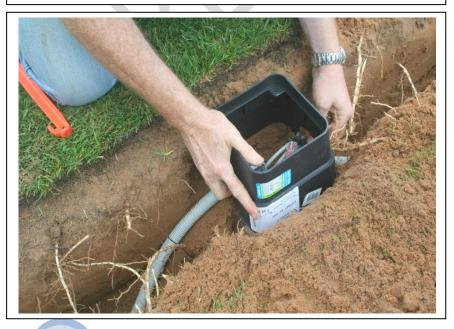
Position a valve box over the cable join.
