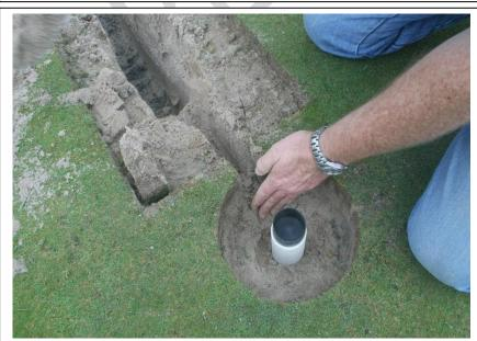
Prepare the probe and cable for installation.
