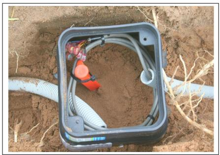
Place cover on valve box and bury to correct height; slightly below ground level.
