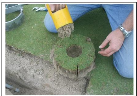
Make a cut on one side to allow for the cable.
