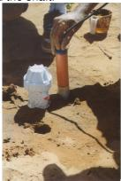
Use a narrow stick to poke around the shaft to remove all the air bubbles.
